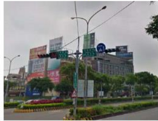
(F)路口纜線及牌面紊亂
